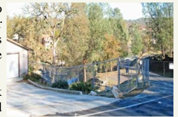
New Kiva Fence Installed
